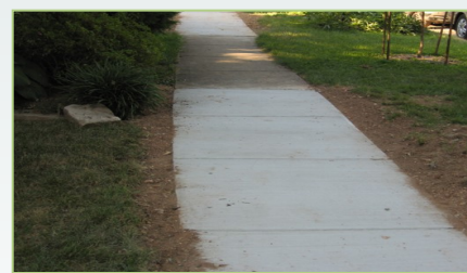
Completed sidewalk repair
